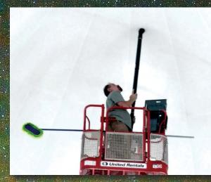
Mark Perkins of Free Fall Technologies of Grand Rapids carefully vacuums the dome to remove dust that has accumulated on the dome and in the finy perforations.
