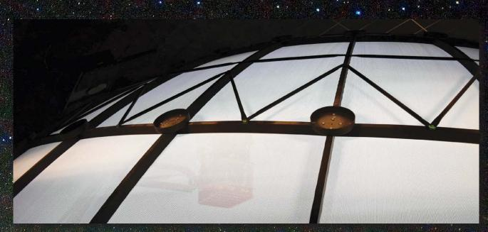
Our planetarium dome is an assembly of 197 perforated panels that contain nearly 7500 tiny holes per square foot. Note that one of the lifts can be seen through those tiny holes from the back side of the dome.
