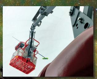
Accessing the upper portions of the dome required the lift to extend nearly 35 feet above the planetarium floor.
